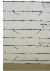
9. Should it be necessary to field cut a panel, which would remove the interlocking fingers, the joint must be tied together. On the two forms you need to connect, every other wire on the bottom 3' and every 3<sup>rd</sup> wire on the top 5' will need to be slid back at least 2 eyelets. Put the forms together and using extra wire that is provided, slide the wire through the eyelets, connecting the forms together. Put a 120 degree bend on both ends of the wire so the forms are secured.
