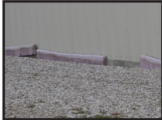
This building only had the insulation installed on the exterior and only went down approximately 1'. You can see that much of the insulation is gone.
