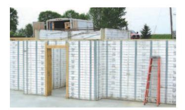
Perma Form does not require special windows or doors. Openings are cut into the forms after they are set and can be made any size.
